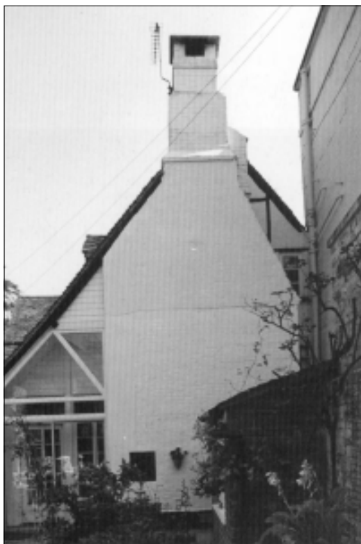
12. Rear of The Tudor Cottage today, showing roof line over conjectural aisle.
