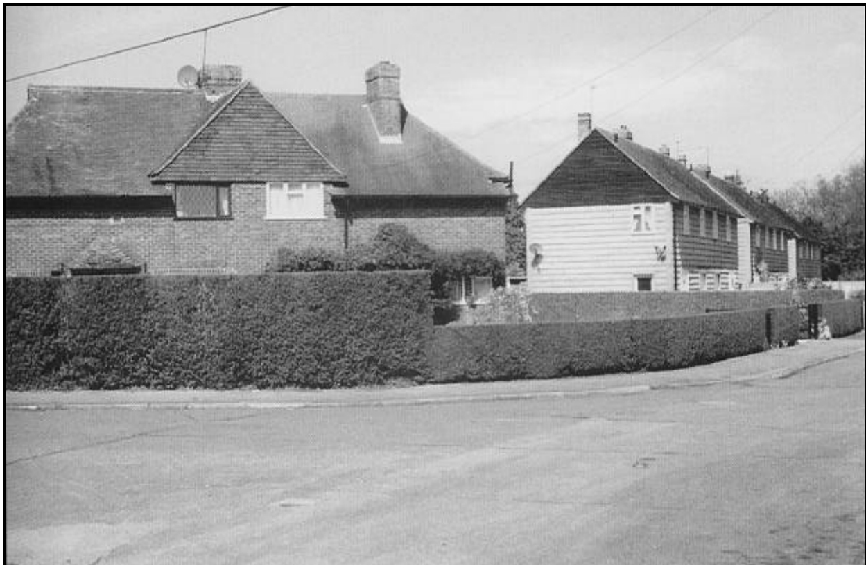
17. Walden Cottages The estate was started by Guildford Council in 1939 and was completed after World War II. This picture shows the two forms of construction of the houses, the Airey Homes on the right and traditional brick-built on the left. Note the beautifully kept hedges. The gardens behind are equally immaculate.
